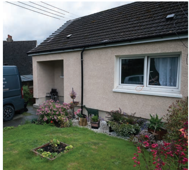
Fig 7. End of terrace house in Argyll and Bute.
