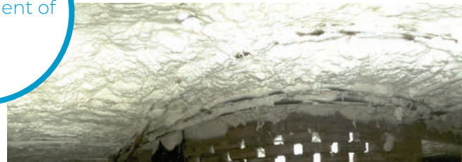
Fig 9. After the installation, showing the insulation now applied.
