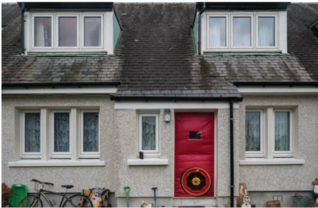
Fig 2. A property in Argyll undergoing airtightness testing.
