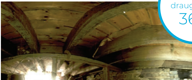
Fig 5. Before the installation.
