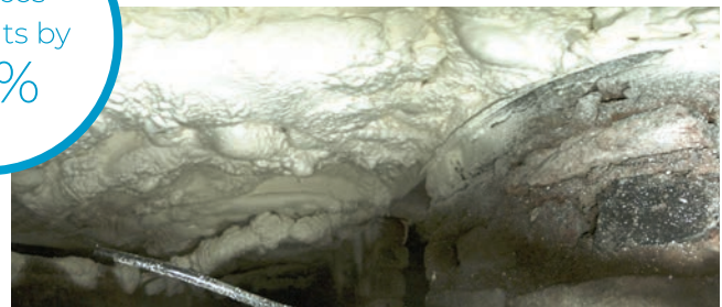
Fig 6. After the installation, showing the insulation now applied.
