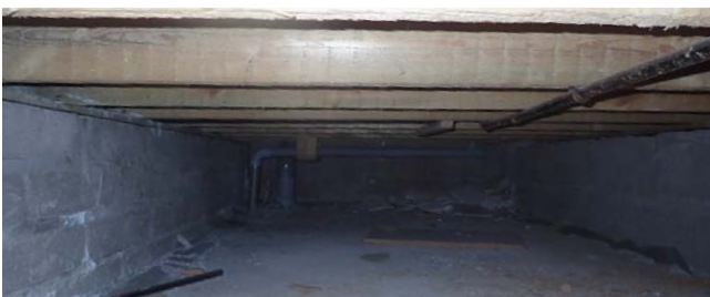
Fig 8. Before the installation.
