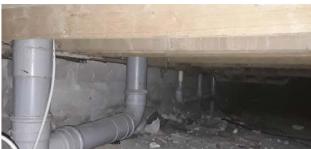
Fig 5. Before the installation.
