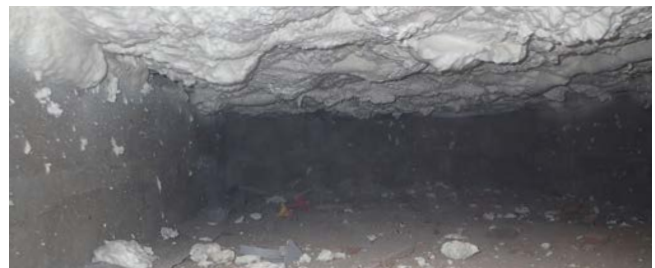
Fig 9. After the installation, showing the insulation now applied.
