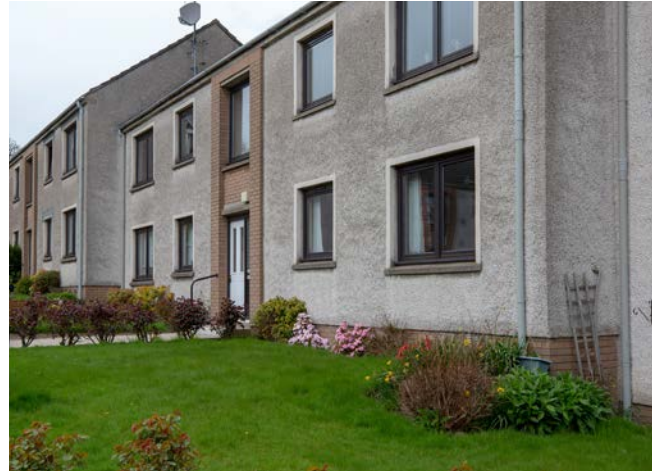
Fig 4. Ground Floor Flat in Aberdeen.
