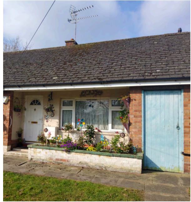
Fig. 3 Entrance of the mid-terraced bungalow.
